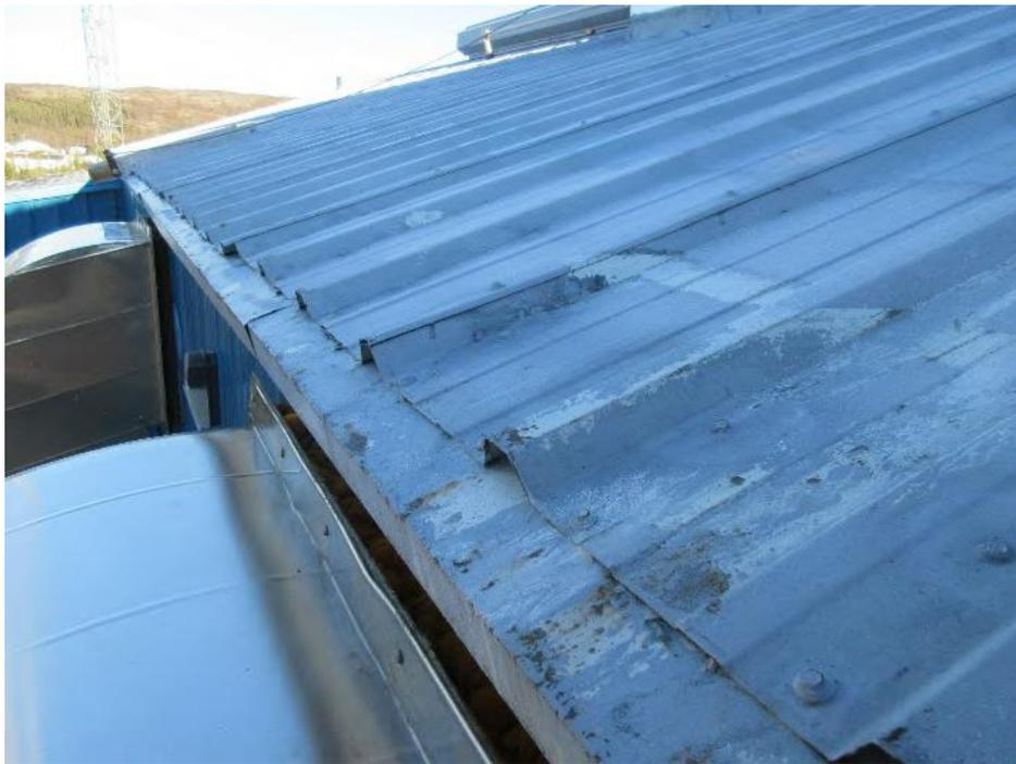
Figure 2: Roof Area where Patching and Sealing has been Attempted.
