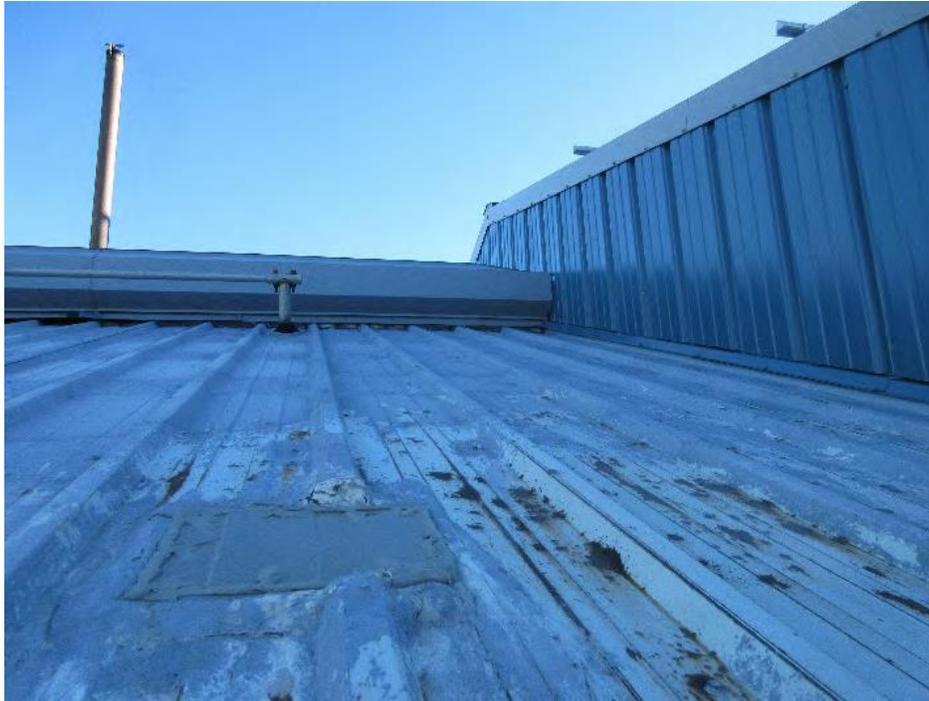
Figure 3: Large Section of Roof with Rusted Panels - Patching/Sealing has been Attempted
