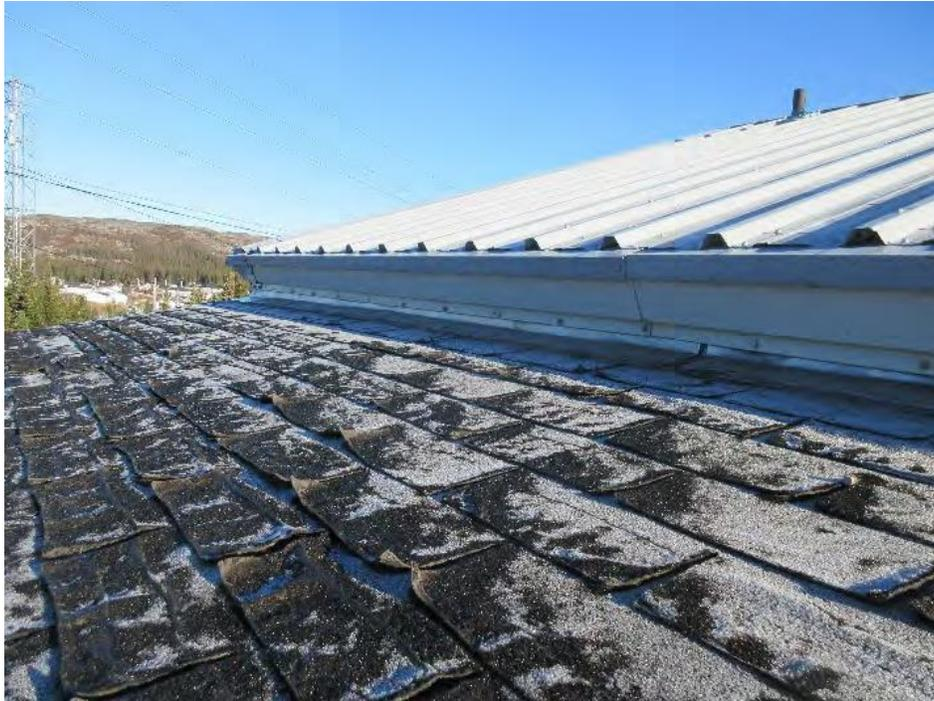
Figure 1: Curled and Cracked Shingles on Storage Room
