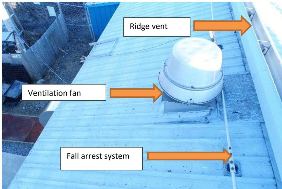
Figure 6: Exhaust Fan Hood (which has been patched around), Fall Arrest System, and Ridge Vent. These Systems are No Longer Required and would be Removed, Reducing the Amount of Roof Penetrations
